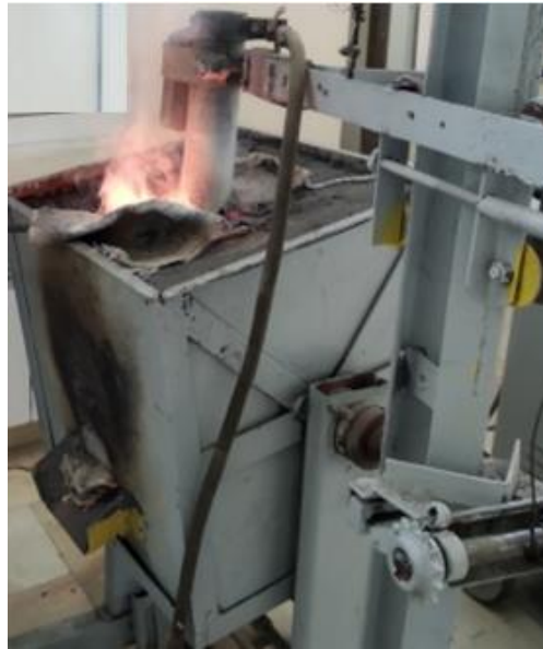
Figure 1. Appearance of electric arc furnace
